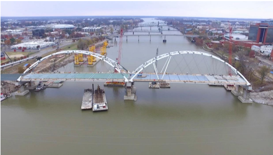
Photo 1 – Bridge Sections floated in place.
