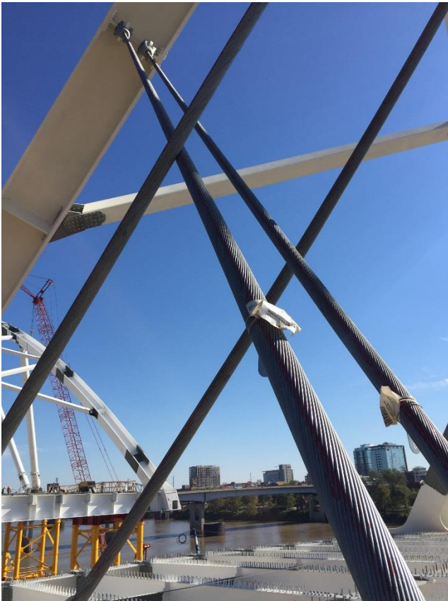
Photo – Installed assemblies.
