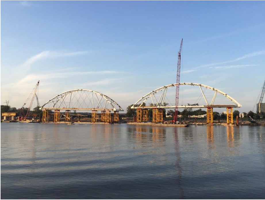
Photo – Bridges constructed on falsework.
