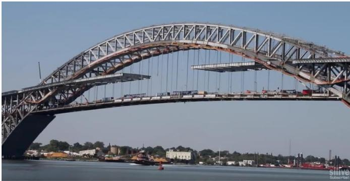
Photo – Bayonne Bridge deck replacement in progress with live traffic.
